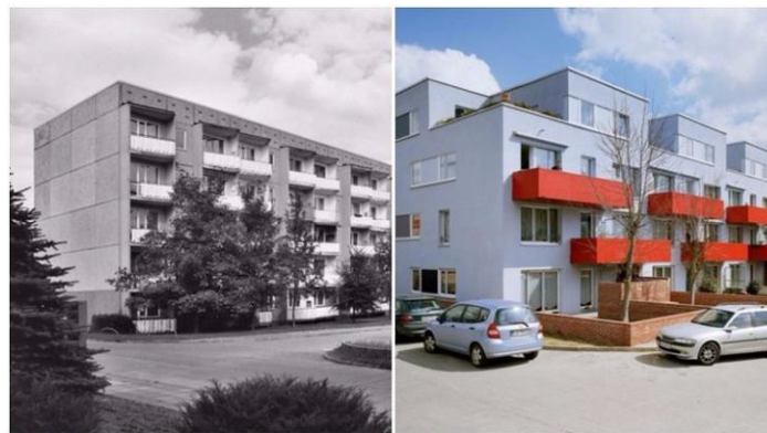
Figure 13. The renovated panel building. Leinefelde-Worbis, Germany
