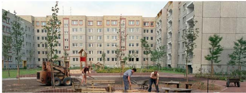
Figure 11. The buildings of WBS 70 series. Magdeburg, Germany
